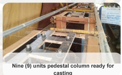
Checking of steel reinforcements and concrete cover (6-16mmØ vertical bars; 10mmØ stirrups spaced at 200mm)
