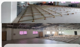
Raised Floor Pedestal and Panel Installation
