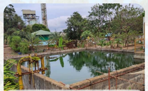
Water Source for Batching Plant 1 and 2 for concreting works
