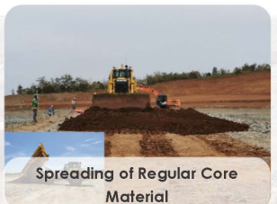
Spreading of Rock Material
