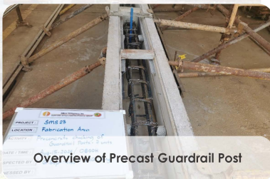
Inspection of rebar works and dimensions
