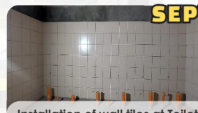
Installation of wall tiles at Toilet areas
