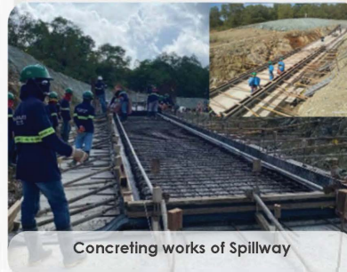
Inspection of rebar and formworks prior to concrete pouring
