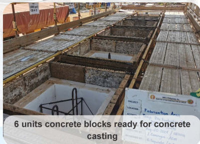
Checking of thermocouple wire locations
