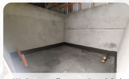
Waterproofing works at 2 nd Floor Toilet
